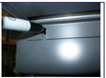
Using the 5/8" self drilling screws provided, start the screws leaving enough room for the solar panel to fit over.
