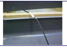
Use the wire clamps provided to secure the wire to the curb. Secure the wire near the top of the curb but not above the curb. From the bottom of the curb run the wire to the right around the corner and up the right side as shown.
