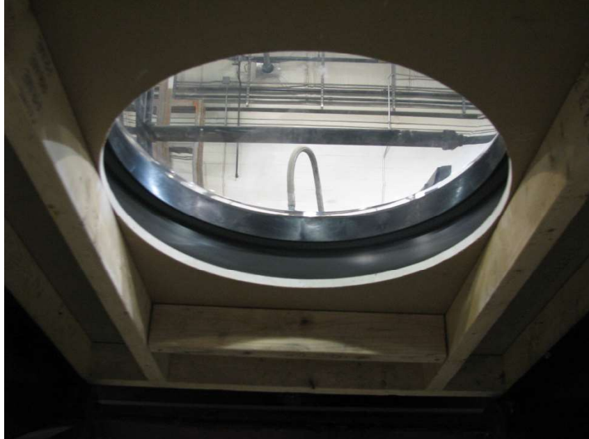
Photo No. 2 Underside of Test Deck (Pre-Test)
