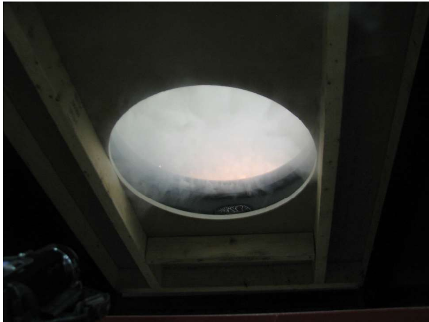
Photo No. 5 Underside of Deck During Brand #1 Exposure
