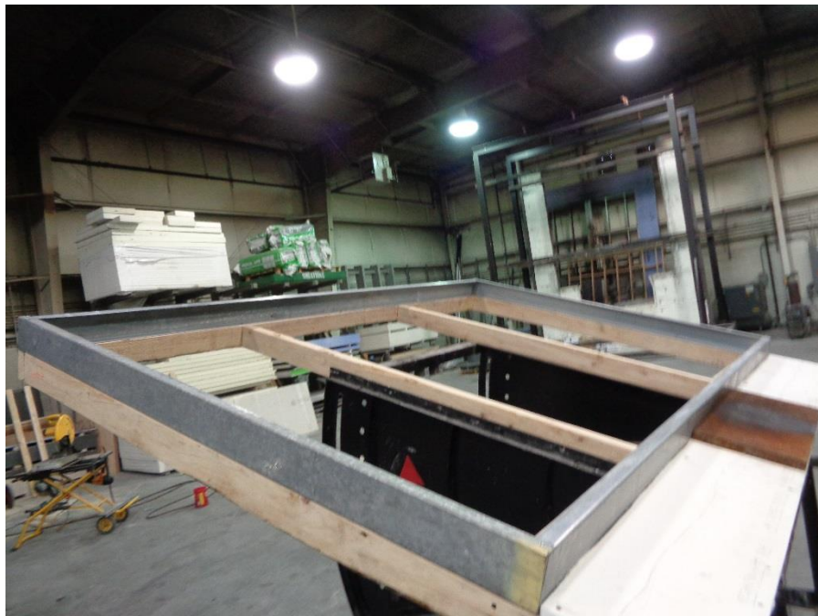
Photo No. 1 Metal Curb Installed to Deck
