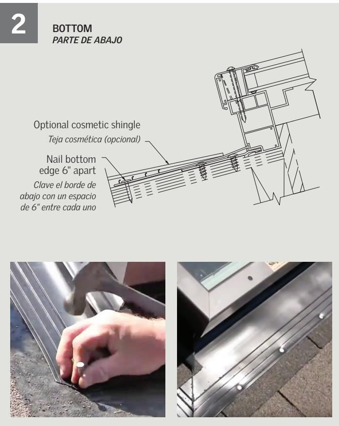
At the bottom: Place flange over shingles and nail the outer edge of the flexible Ultraseal Flashing down to the roof deck with roofing nails spaced about 6" apart. Then apply one nail to each top corner to hold unit in place. Ultraseal Flashing is self-sealing around nail penetrations.
