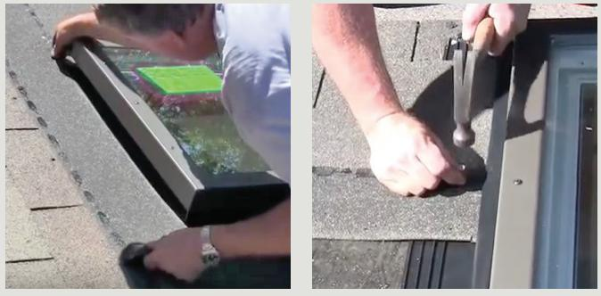
At the sides: Place shingles over flat ribbed portion of flexible flange, then trim shingles as needed, and tuck UNDER L-Gasket and nail.
