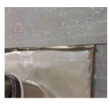
Position the base roofing material or felt over the folded top edge of the tile flashing, stopping short of the vertical fold.
