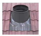
**49 CAUTION:** Do not penetrate the flashing with the tile fasteners.
