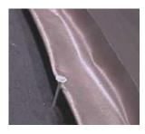
9 Bend 1" of the folded edge upward. Secure in place with roofing nails. **CAUTION:** Do not penetrate the flashing with roofing nails.
