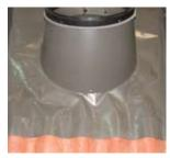
Form the bottom of the tile flashing to the contour of the tiles.
