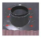
Secure the standard VELUX SUN TUNNEL™ skylight flashing to the roof deck with the screws provided.
