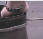
6 Install the intermediate ring to the top of the tile flashing. Secure with screws. The condensation weep channel can be used to seat the two alignment notches.
