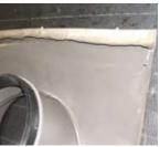
Any water that makes contact with the base roofing material should flow around the tile flashing; therefore, the side water diverter must be flattened to create the top diverter.
