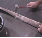
8 Create the top water diverter by folding 3" to 4" of the tile flashing top edge back on itself. Then flatten.
