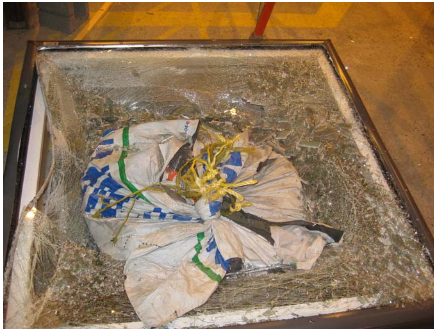
Photo No. 2 Damage from 1600 lbf Drop at 8'
